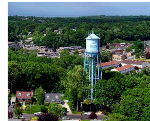
Glen Cove Water Tower Image: Nestor Rivera
