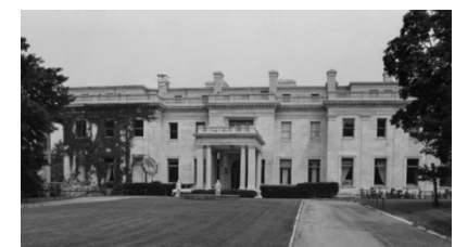
Winfield Hall, Woolworth Estate
